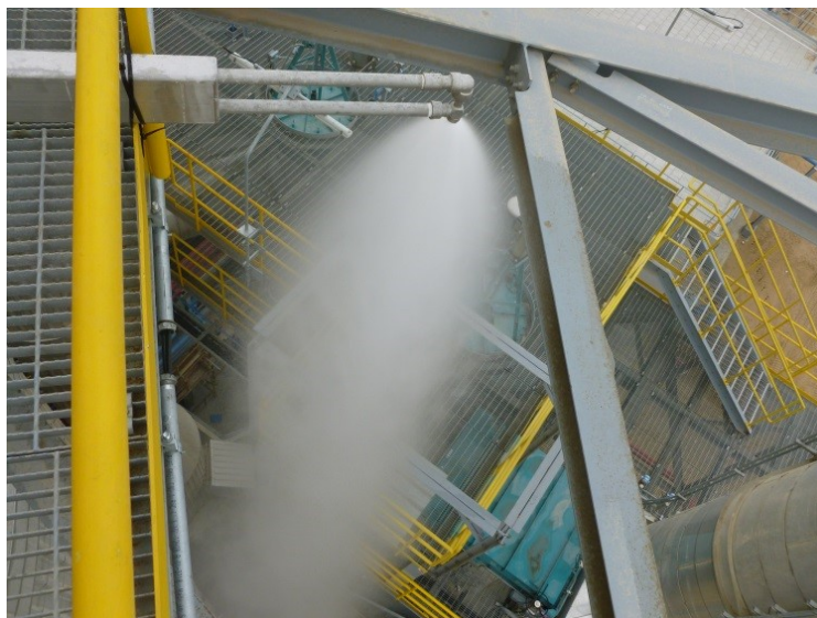
Figure 4. Inspection of lance spray with correct pattern.
